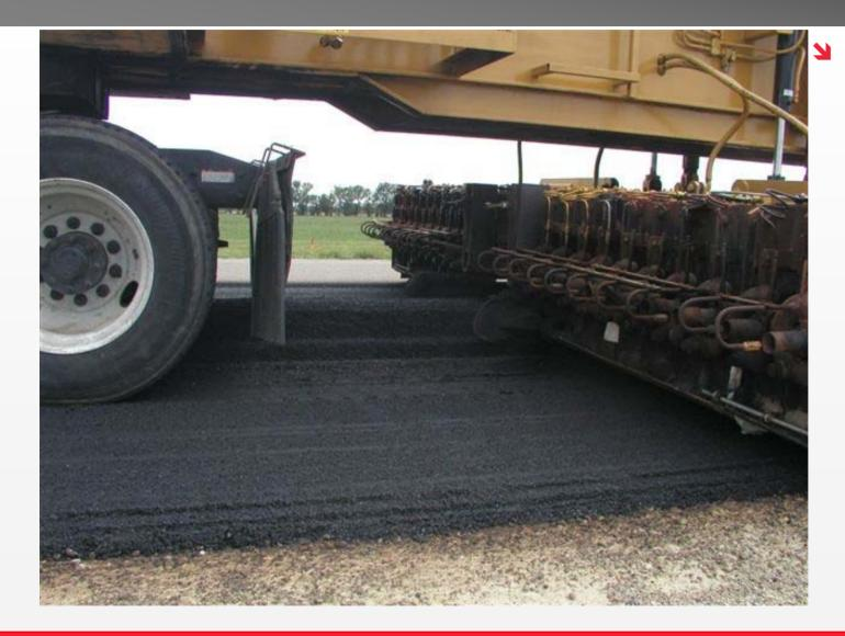
Heated, Milled Windrow Going Through Tunnel Heaters
