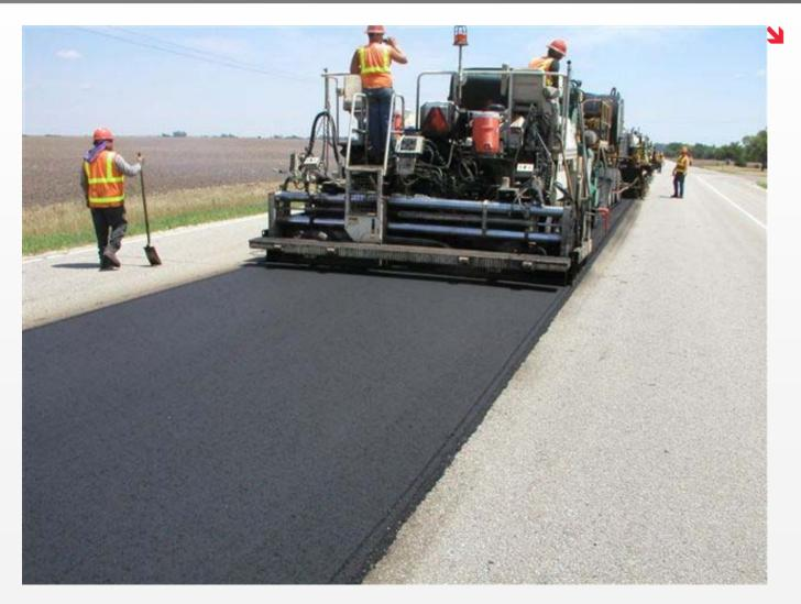
Recycled Asphalt Mix Placed with Paver and Vibratory Screed
